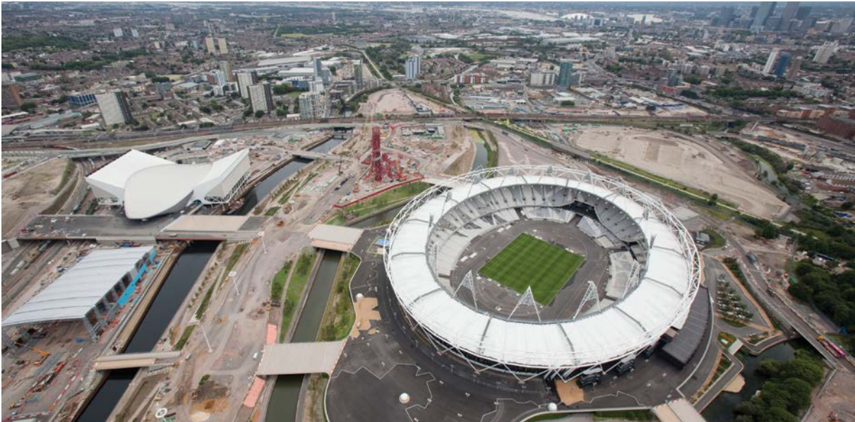
Fig 1.1 Aerial view of the Olympic Stadium during development. Courtesy of London 2012, © ODA 2008.
