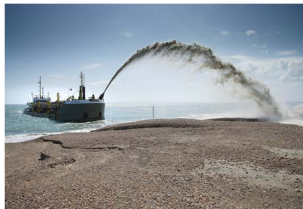
Fig 1.2 Pumping material onshore, © Westminster Dredging Company Limited.
