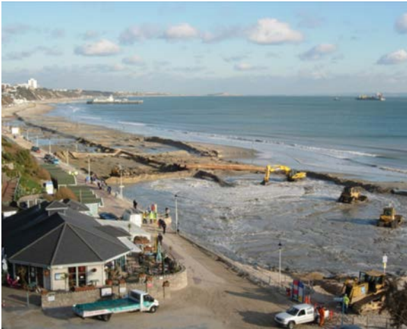
Fig 1.3 Coastal defence works under way, © Westminster Dredging Company Limited.
